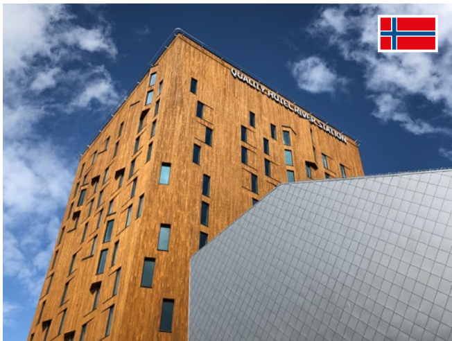
Quality Hotel Rivers Station, Drammen
