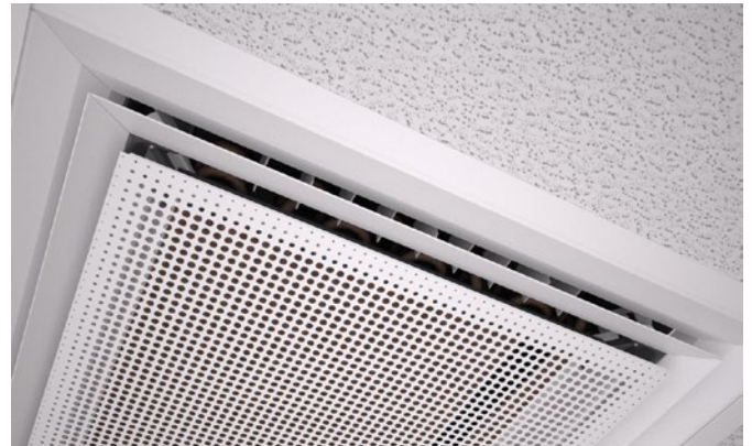
Figure 12. PD face plate Circular holes arranged in a square pattern with a graduated border
