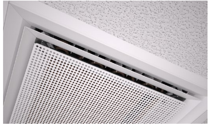
Figure 11. Standard face plate Circular holes arranged in a square pattern
